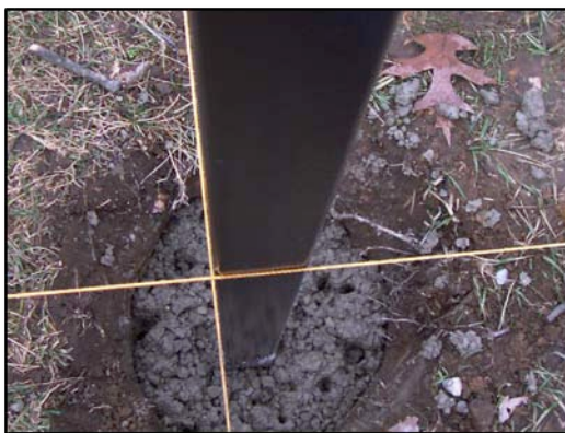
Figure 6 - Post Hole Should be Positioned so That The Centered Post Will Contact Your String Line
