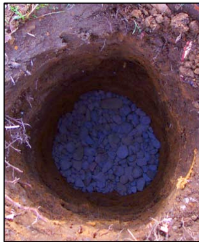
Figure 7 - Adding Gravel to the Bottom of the Hole is Not Required, but Can Be Beneficial
