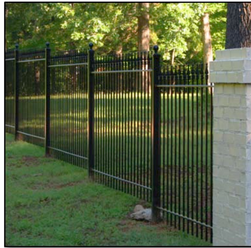
Figure 13 - Stair Stepped Fence Panels
